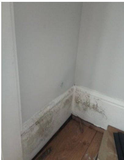
Sunken floor repaired and damp in dining room
